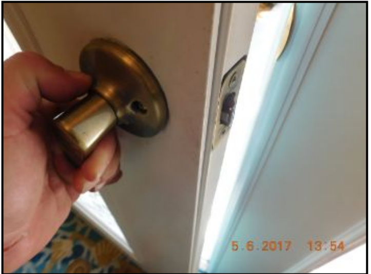
Push button does not go in all the way and sticks in the catch plate
