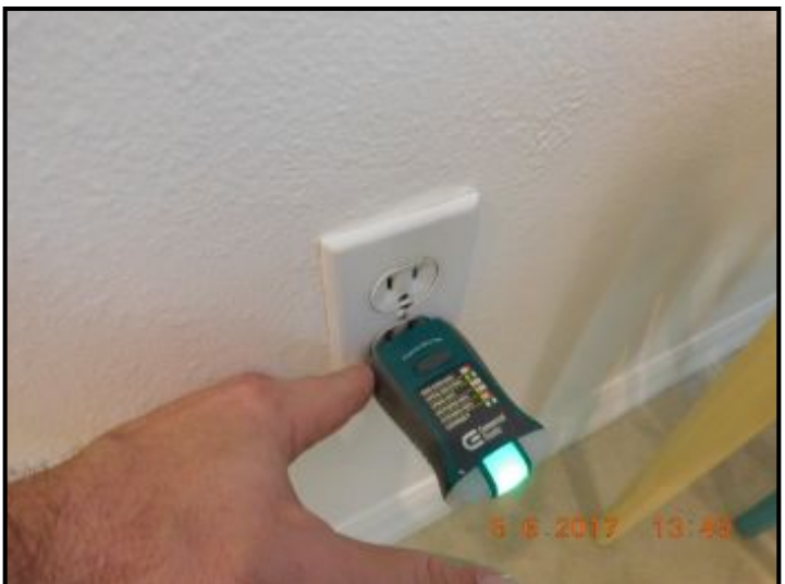
Outlet is loose in the wall
