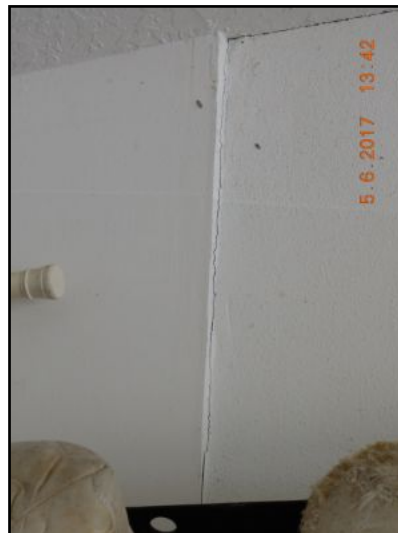
Drywall separation noted on interior garage wall
