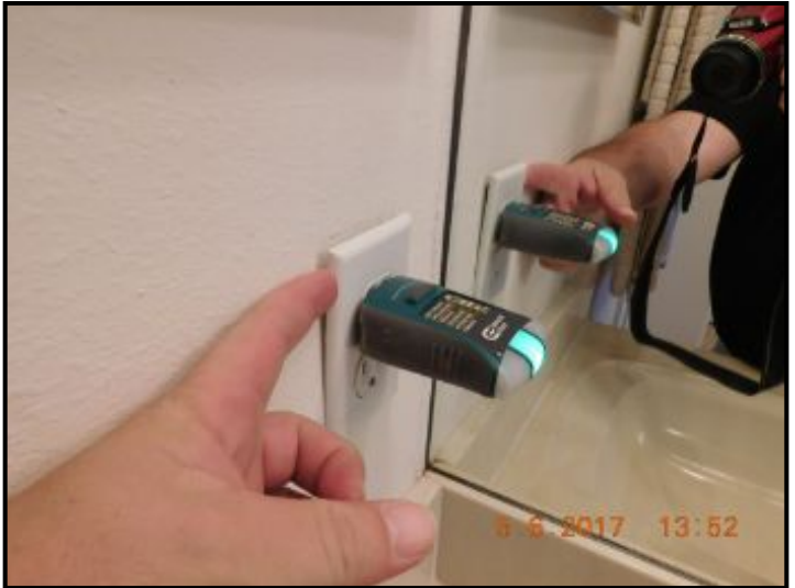
Outlet is loose in the wall
