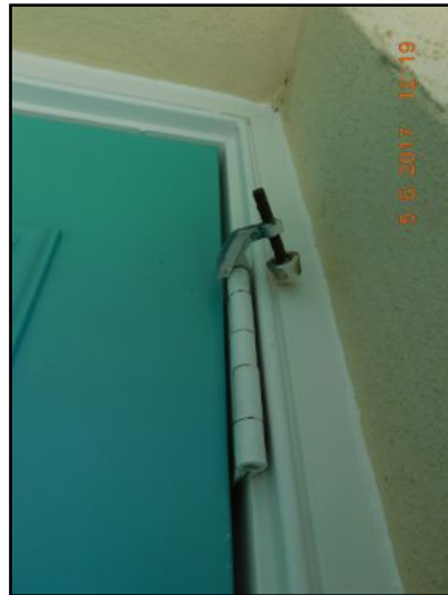
Door stopper is bent
