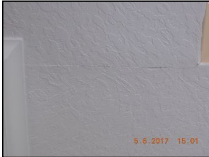
Drywall tape separation noted between entry way and kitchen
