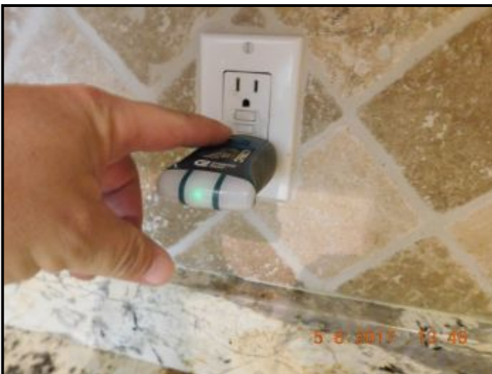
Other outlets with GFCI protection are reset at this outlet
