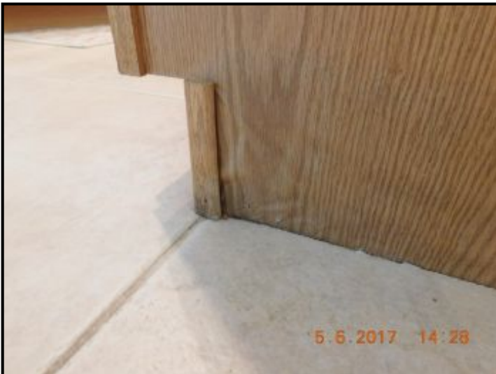
Laminate is peeling away from the cabinet frame
