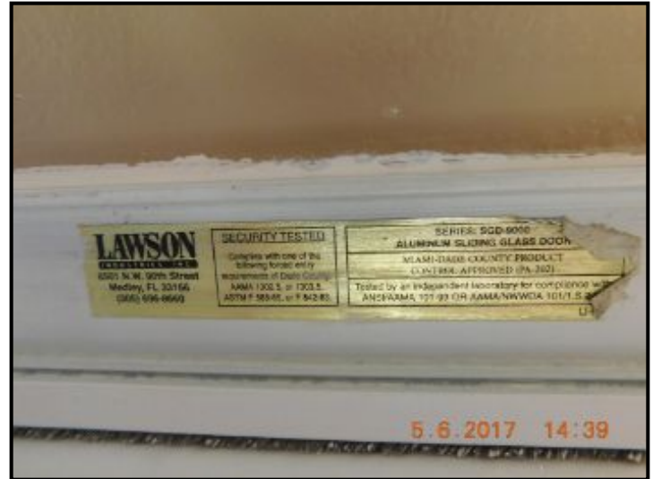
Manufacturer's label on the patio doors, not an impact resistant product
