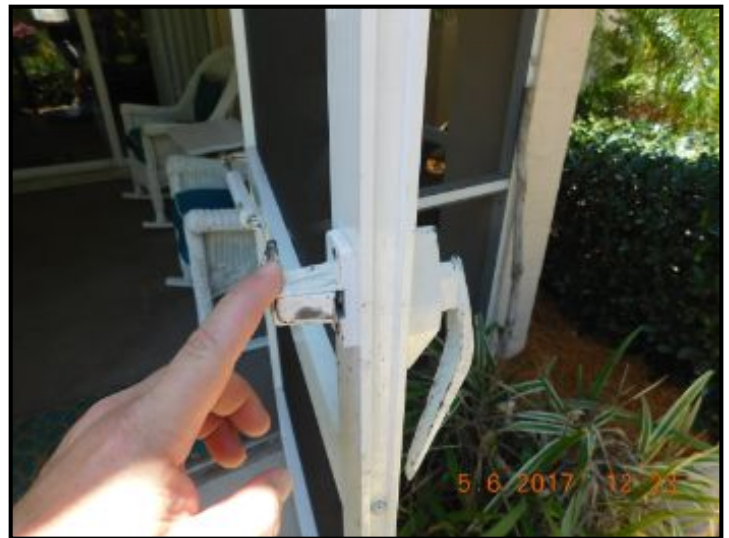
Handle does not close properly
