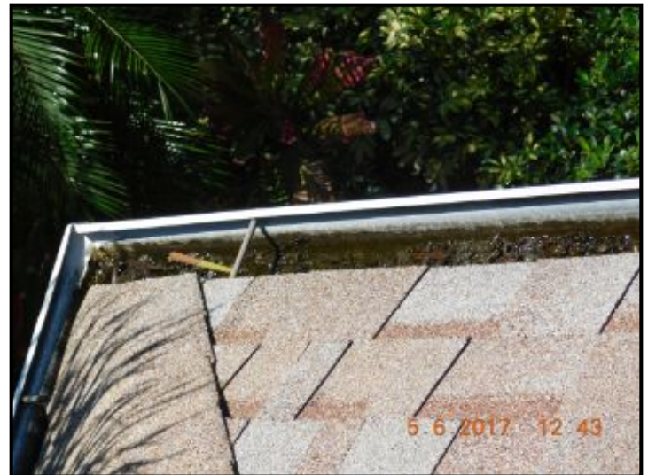
Gutter has a large amount of debris built up above the front entry door
