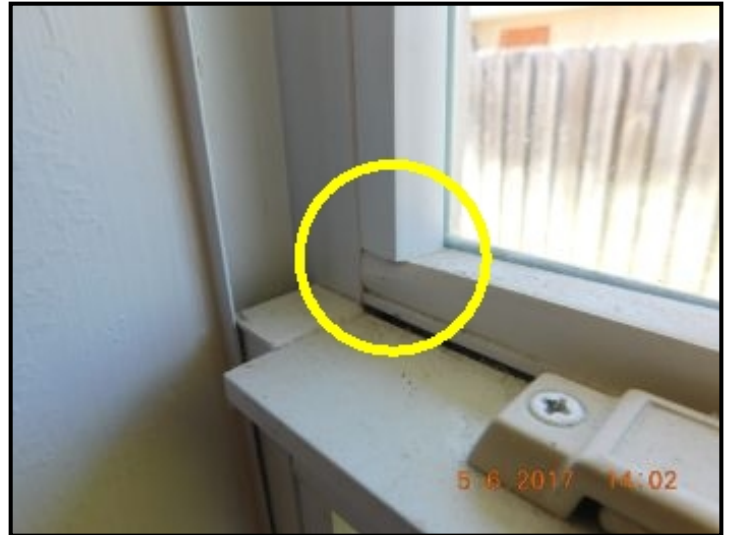
Window catches on the plastic frame when trying to open it
