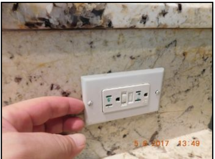
Reset button for GFCI protection is loose
