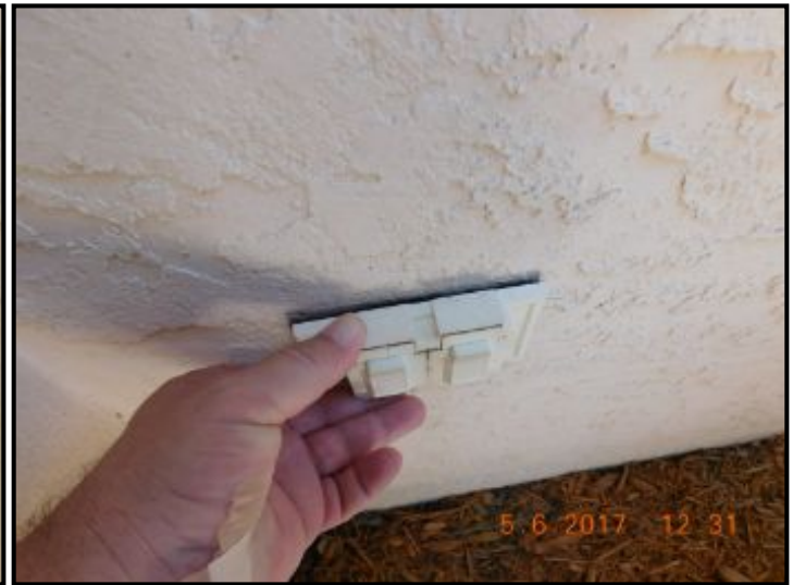
Outlet and plate are loose on the wall
