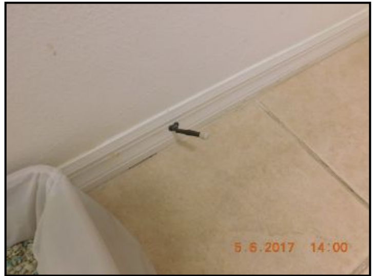
Door stopper is bent
