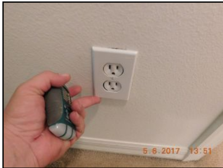
Outlet is loose in the wall
