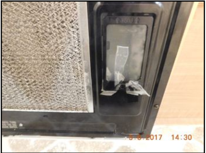
Light does not work and the cover is damaged
