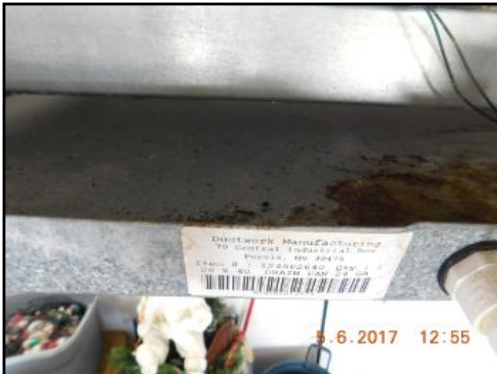
Corrosion noted inside the drip pan
