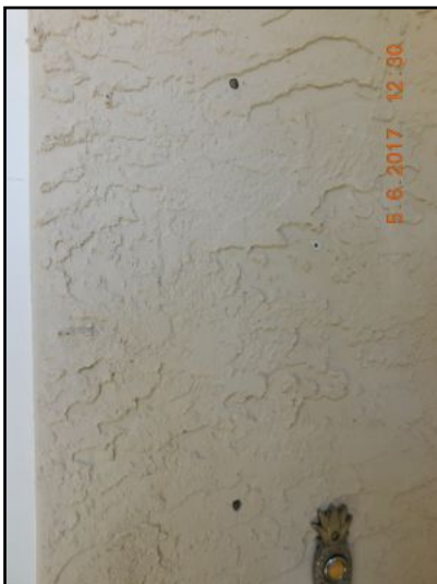
Holes drilled for plywood installation as storm panel protection
