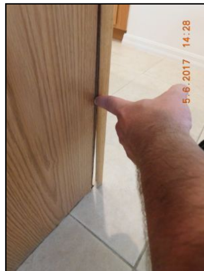
Moulding is loose on the cabinet frame
