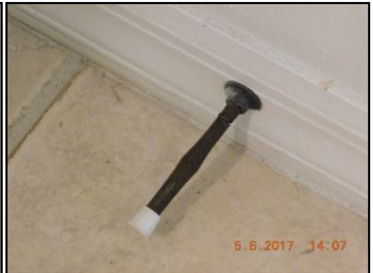
Door stopper is bent
