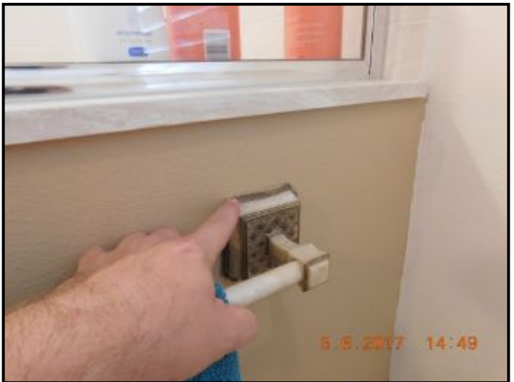
Tower bar is loose on the wall
