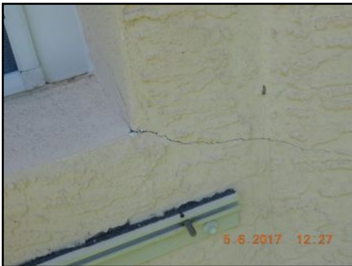
Minor settlement crack noted below the window
